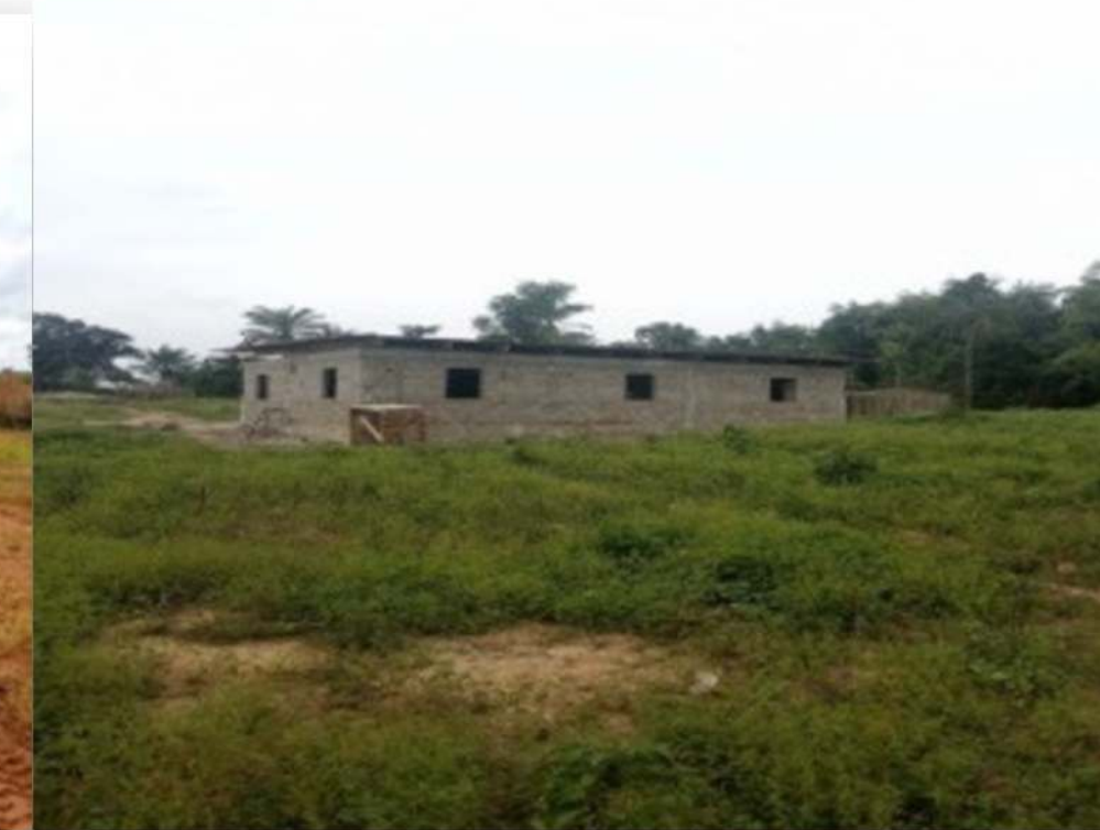
Medical Clinic Construction
