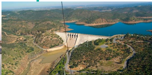
Andevalo Hydroelectric/Water Dam
