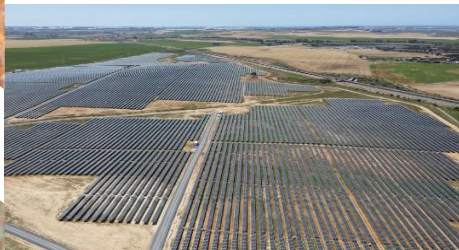
Paymogo Solar Power Plant
