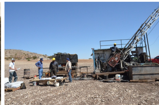
Drill Rig – Site Visit 2012
