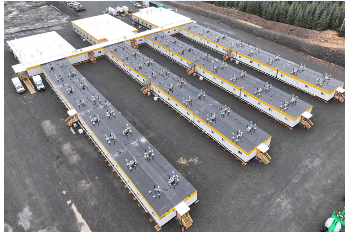
CAMP 11 WORK AREA
